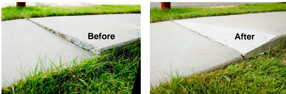
Figure 10: Precision Sidewalk Safety Work Example
